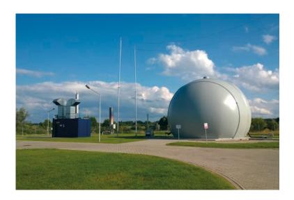
TEDOM Poland commissioned a containerized CHP unit Cento T100 at the wastewater treatment plant in Morag, Poland in June 2015. The CHP unit covers the energy needs of the WWTP and in case of distribution network failure, it can also serve as an emergency source of electricity and heat to maintain the operability of the wastewater treatment plant technology.
